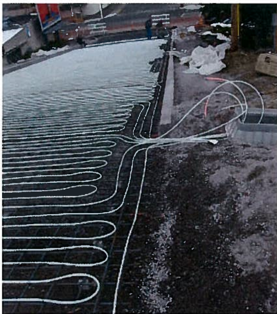
Figure 6. The approach road loops placed latitudinally.
