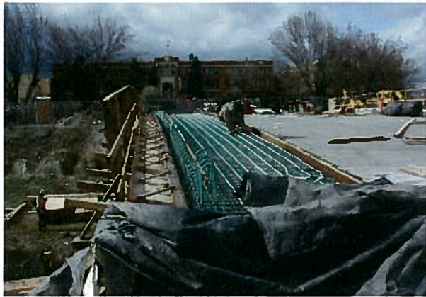
Figure 5. Bridge sidewalk loops.
